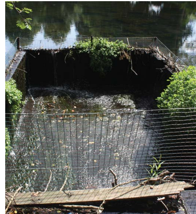
Outlet in north lake
