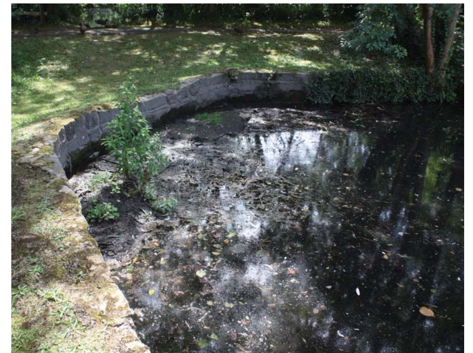
Excessive silt material within the south east corner of Lake 4
